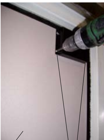
Door Panel Attach Cover Plate Over Hinge With Screws
