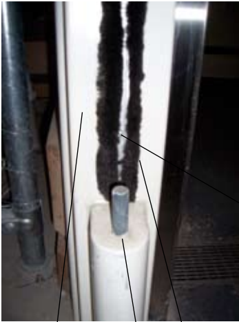
Door Frame Pivot & Guard Brush Seal
