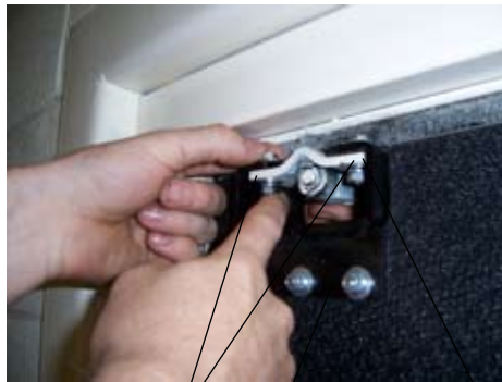
Attach Bolt Nut & Washers Top Hinge Top Hinge Pivot Plate
