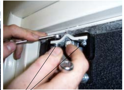
Tighten Up Nuts & Bolts Centre & Align Door Panel
