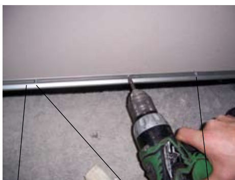
Brush Seals Attach Brush Seals With Screws
